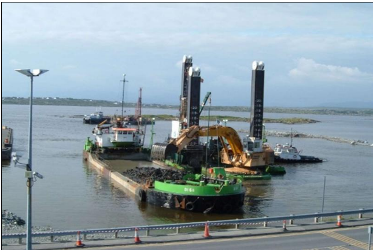
Figure 3-8: Backhoe Dredger Loading a Barge
