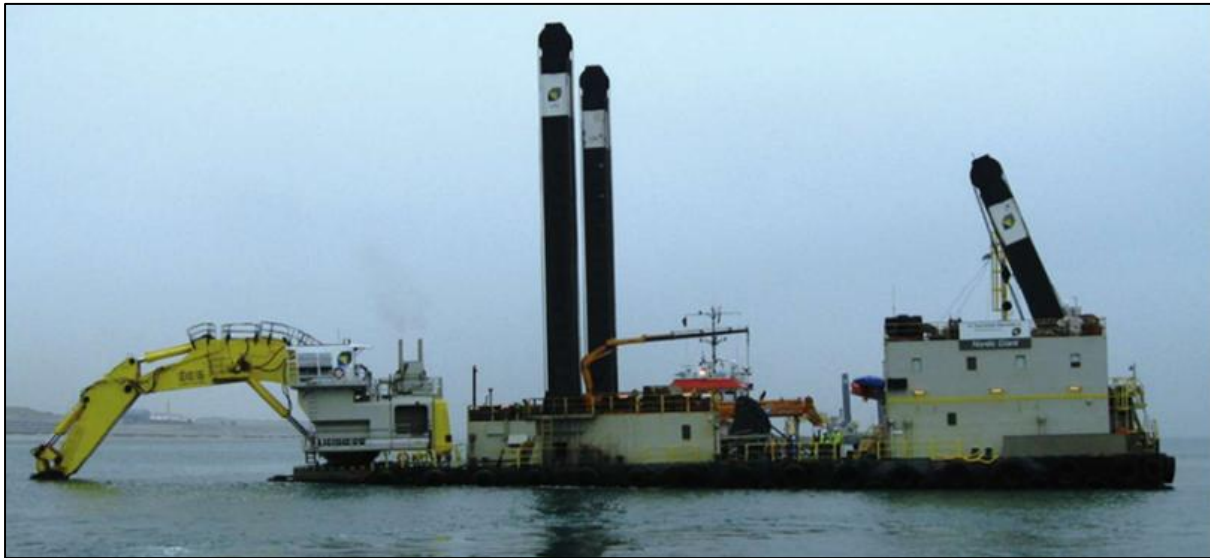
Figure 3-7: Backhoe Dredger in Operation
