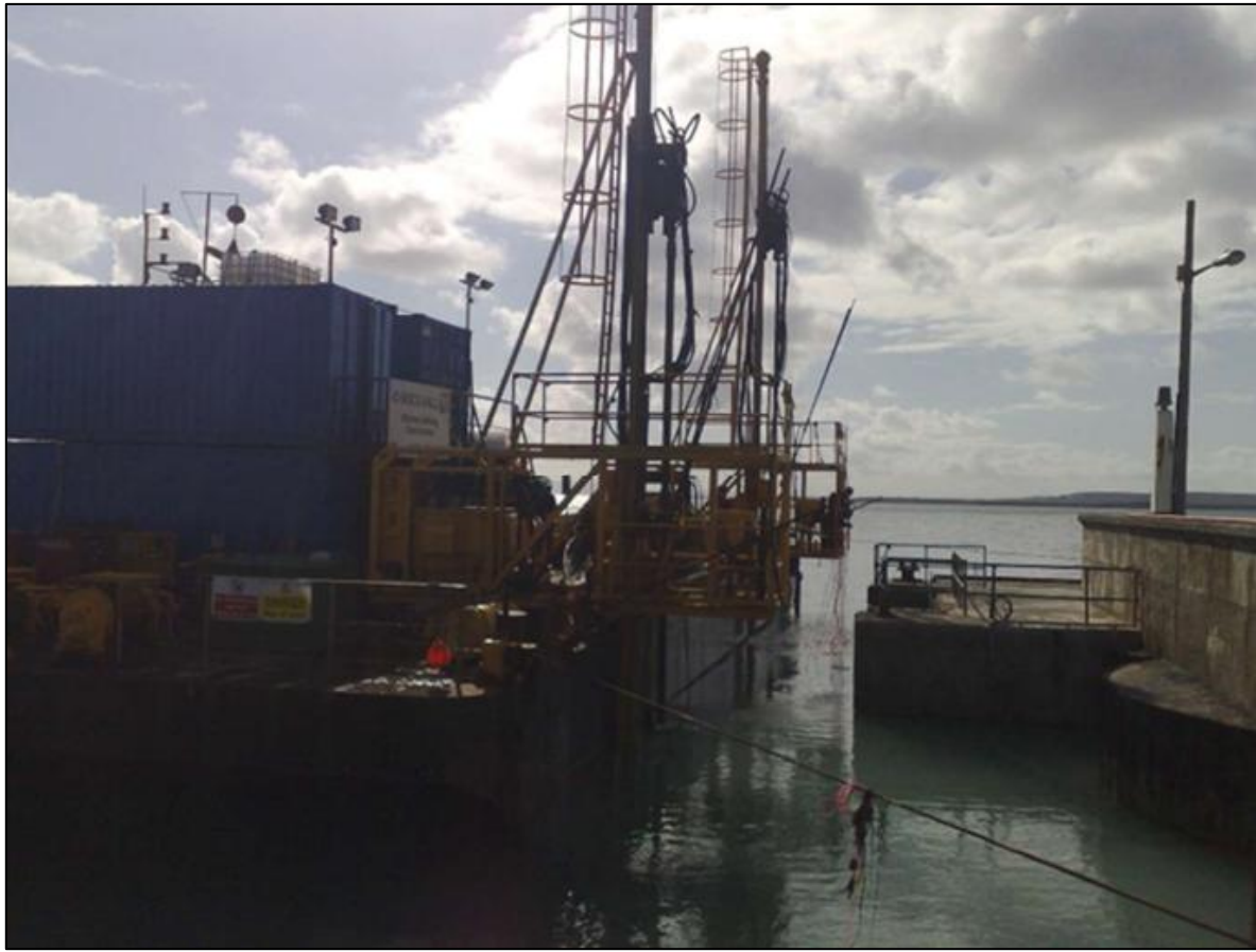
Figure 3-6: Pontoon with Two Drill Rigs
